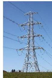
dead-end tower (anchor pylon, 3D truss)
