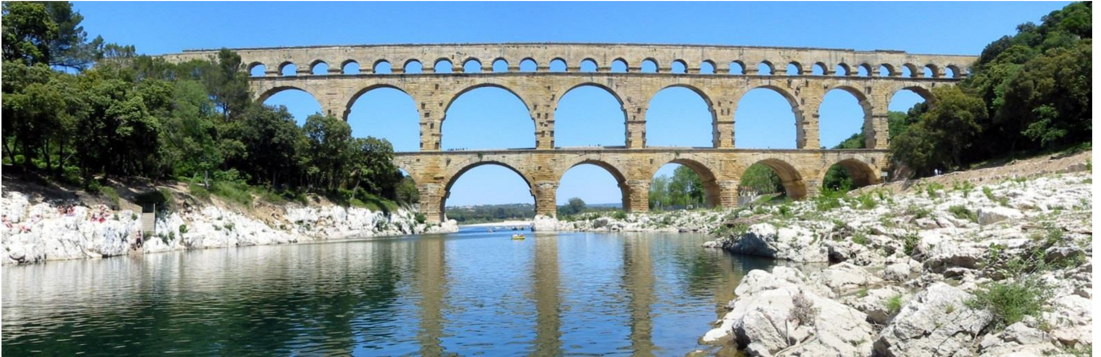
Roman aqueduct, an example of an arcade, employing the circular arch
